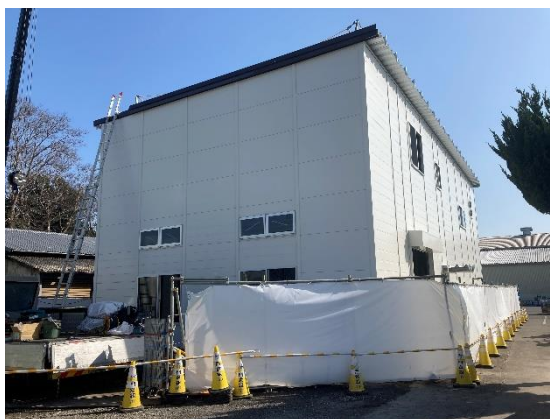
Information Center under construction (photographed on March 15, 2022)
